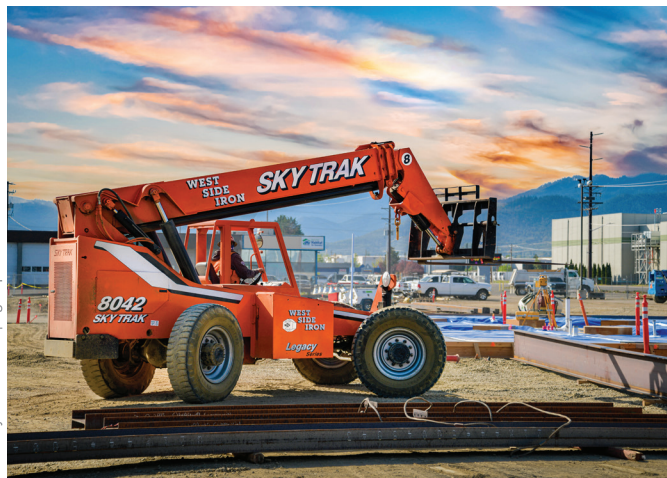
A telehandler at an S&B James Construction worksite
